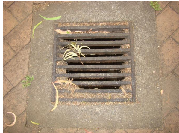
Plate 10. Subsurface services in central courtyard of southern lot.
