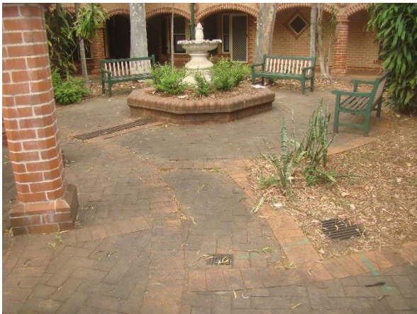
Plate 9. Subsurface services in central courtyard of southern lot.
